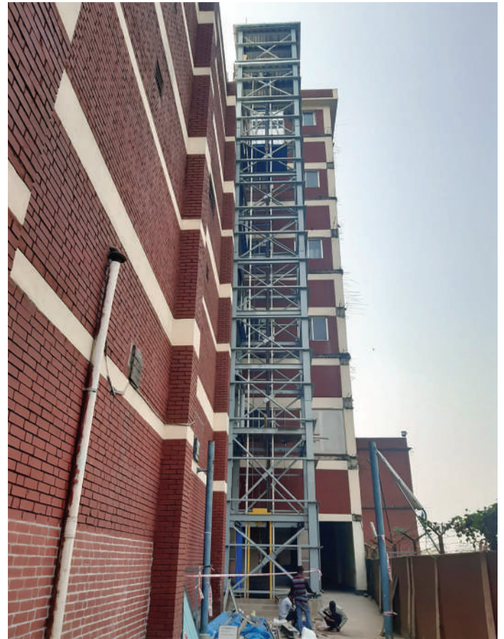
STEEL LIFT CORE (JMI GROUP)
