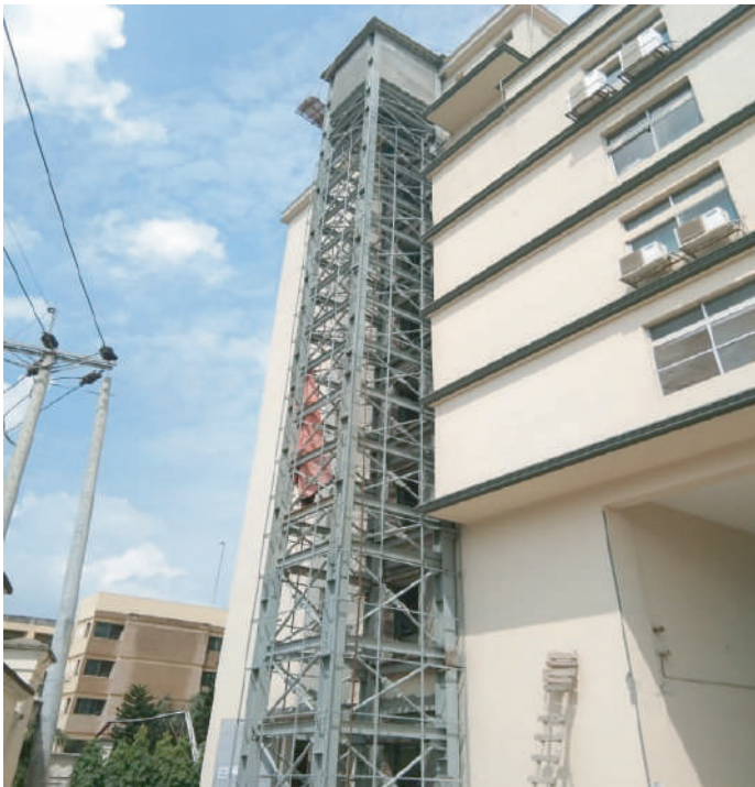
STEEL CARGO LIFT CORE DURING WORK (SILVER LINE COMPOSITE TEXTILE MILLS LTD. UNIT-1)
