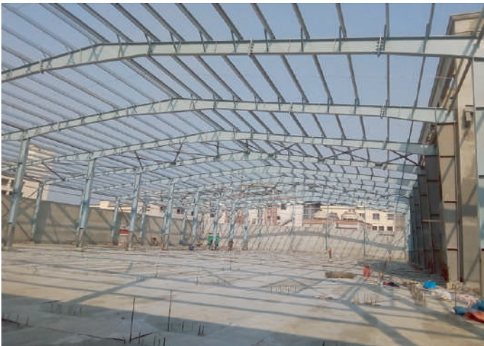
STEEL SHED BUILDING (SPINNING UNIT) DURING WORK (SILVER LINE COMPOSITE TEXTILE MILLS LTD.)
