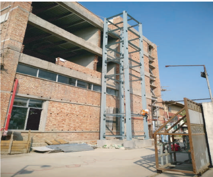
STEEL LIFT CORE DURING WORK (AKH KNITTING & DYEING LTD.)
