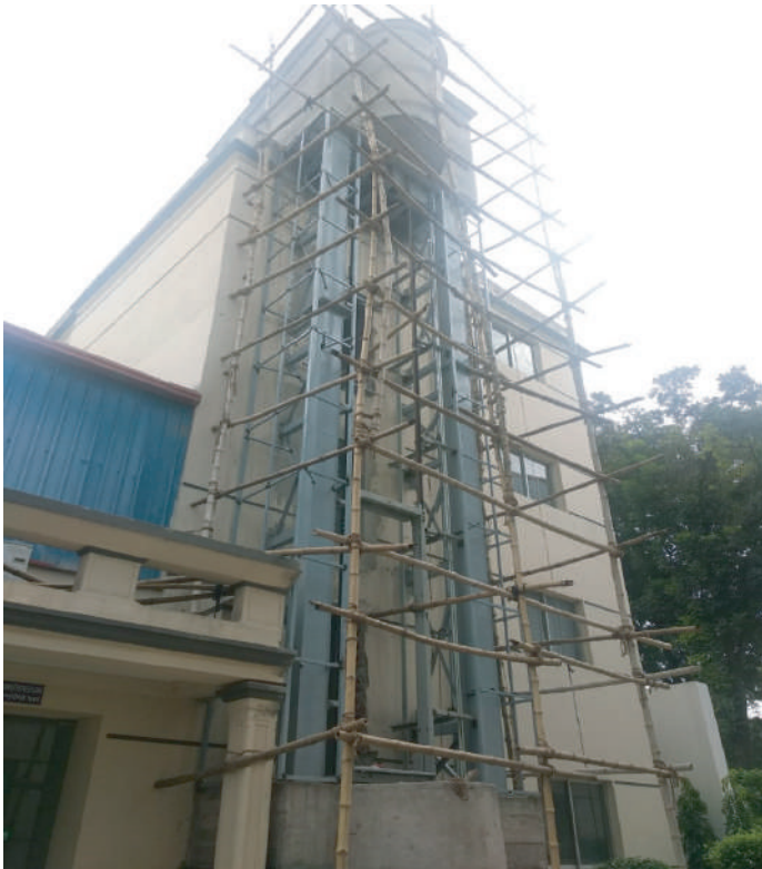
STEEL PANORAMIC LIFT CORE DURING WORK (SILVER LINE COMPOSITE TEXTILE MILLS LTD. UNIT-3)
