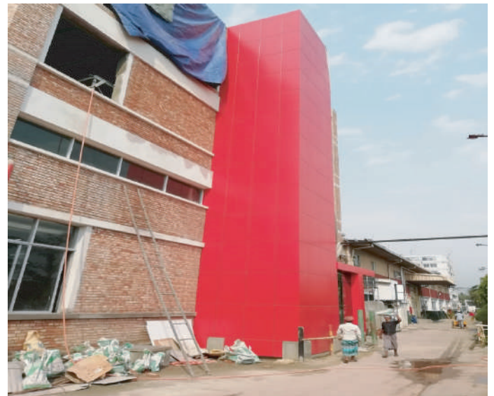
STEEL LIFT CORE AFTER WORK (AKH KNITTING & DYEING LTD.)
